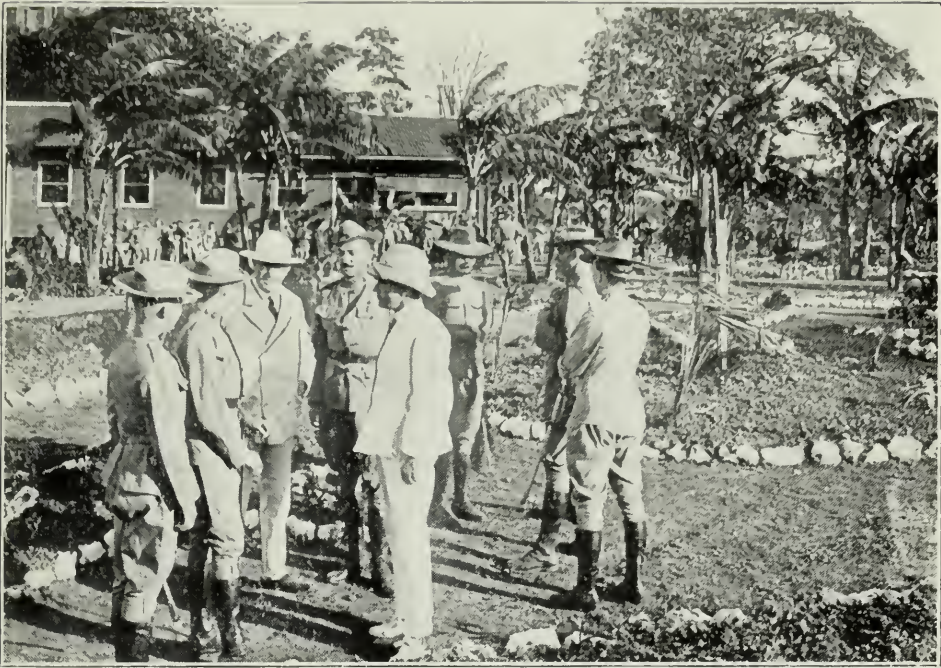
MR. BOYCE AT CAMP ELLIOTT, PANAMA CANAL ZONE.
